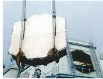
Phased Array Radar ( No moving parts )
